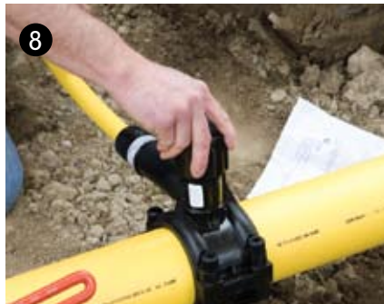
8 Install PMT PermaTite® cap, hand tightening until cap comes in contact with built in stop on tower.
