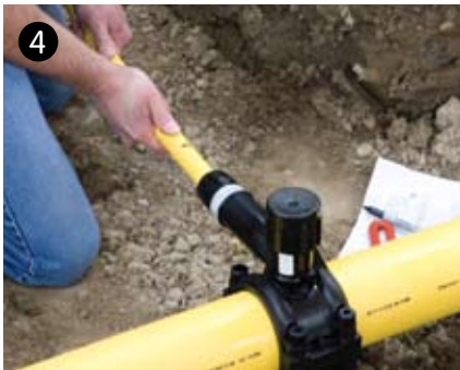
4 Connect service piping to PermaLock tee outlet.
