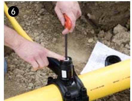
6 Thread cutter downward until the cutter bottoms in the tower. The depth tube is a visual guide and will be approximately flush with the top of the tower when the cutter is engaged.
