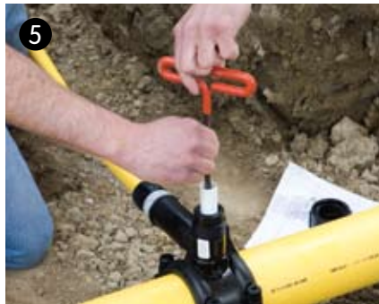
5 Place depth tube on top of cutter assembly.
