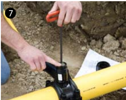
7 Thread cutter upward until cutter is flush with top of tee tower. Discard depth tube.
