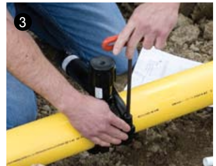
3 Bolt tee onto main until tee tower/base corners touch. The bolt should be flush with the bottom of the base. Stop, do not tighten further.
