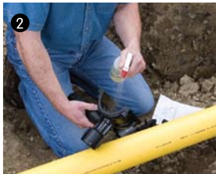
2 Lubricate tower o-ring and surface of main where tee is to be installed.
